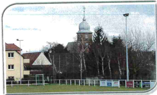
ECLAIRAGE TERRAIN DE FOOTBALL
